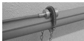
**Attention!** During assembly ensure that the spring may not bounce, as this may result in eye injuries. Should the pipes be covered by insulation material, remove the material from the intended point or mount the temperature probe below.
